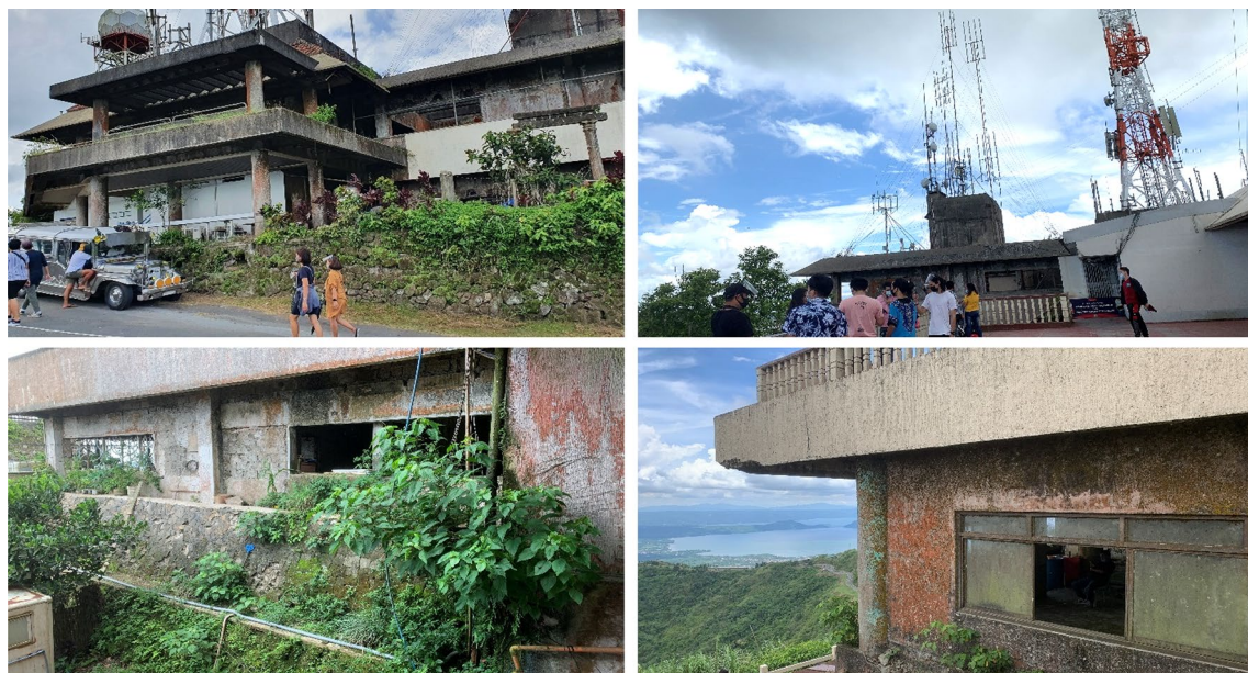
Fig. 10 From left, the neglected annex buildings; several rooftop communications towers; overgrown plants by the lower level; damaged slab and corroded exterior of the annex (Source: Author, 2021)
