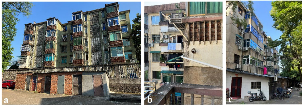
Fig. 15 Unplanned extension: balcony (a), filling (b), ground level (c). Tong, Sujun and Yurong Ling. Exterior of the 1980s' apartments. June 9, 2023
