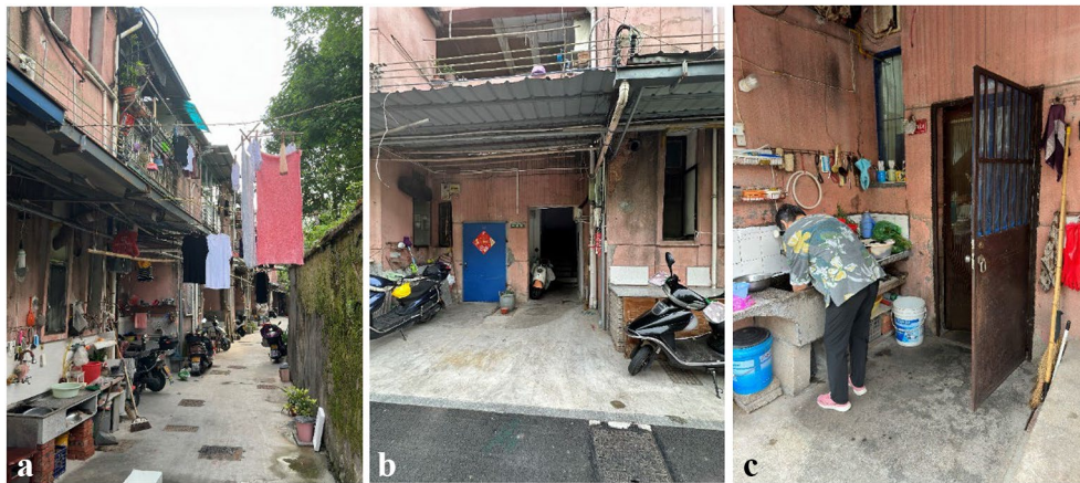
Fig. 27 Unplanned extension: corridor (a), entrance (b), and laundry space (c). Tong, Sujun and Yurong Ling. Exterior of the former warehouses. June 9, 2023
